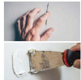
We will inspect any shrinkage cracks measuring over 3mm (width of a pound coin) as part of our two-year warranty, at your request.
