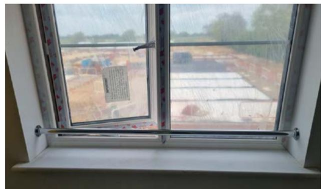
Figure 1: Example of a Part O compliant guard rail
